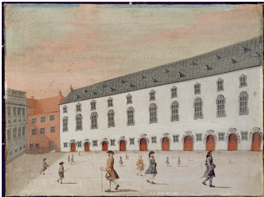
Fig. 2. Kunstkammer building, c. mid-18th century. Painting by Johannes Rach and Heinrich Eegberg, c. 1748–1750
