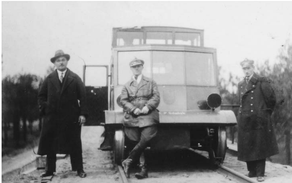
Fig. 6. On control of the Śląsk–Gdynia railway line, 1932
