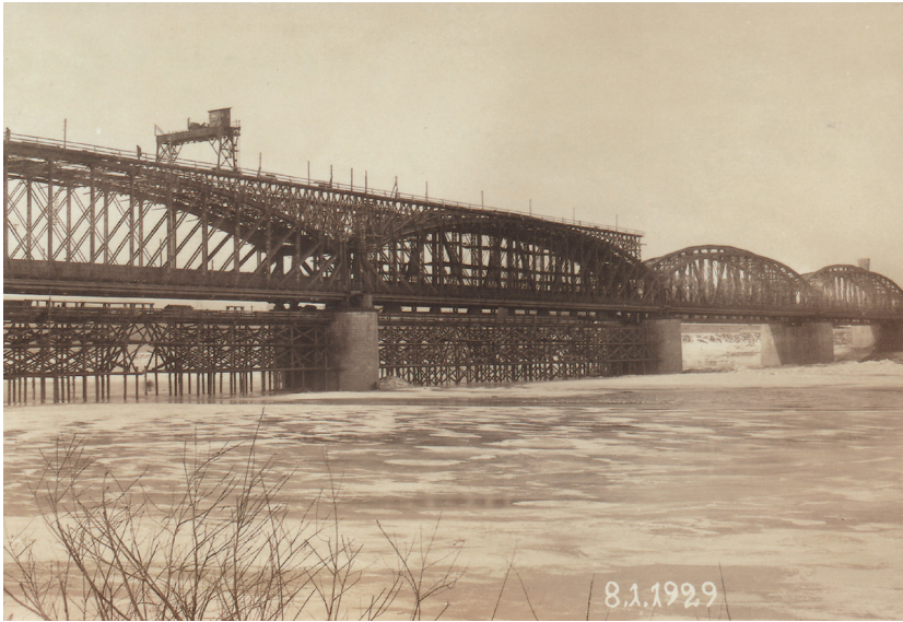
Fig. 4. Toruń railway bridge strengthening, 1929
