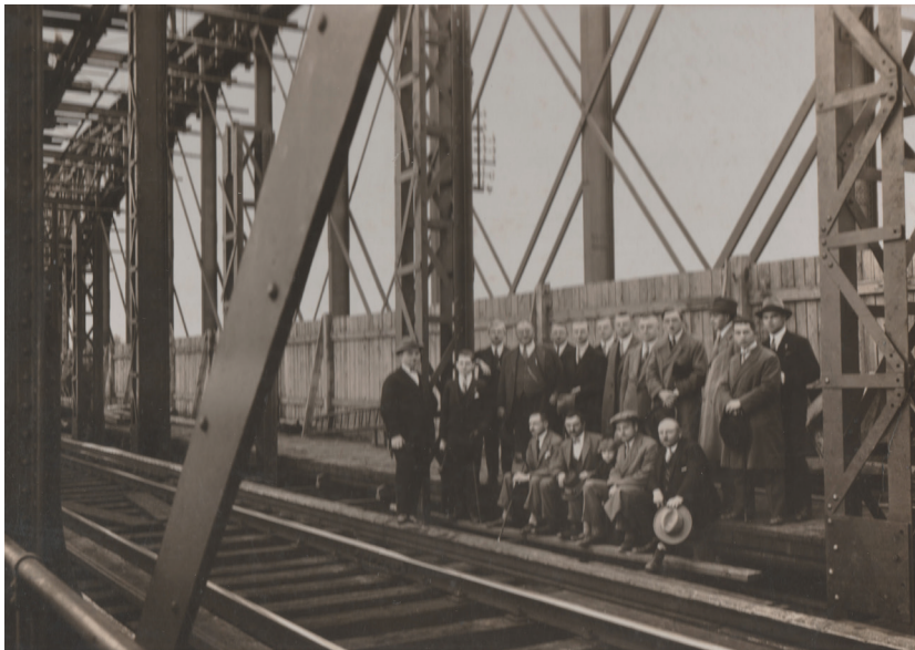
Fig. 5. Bridge rail track terminated, 1929
