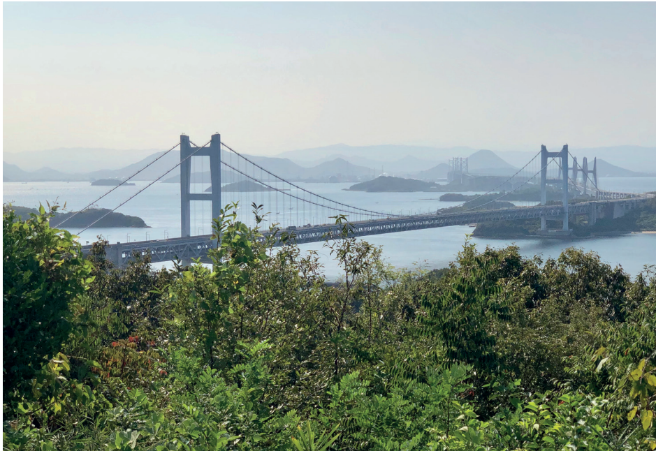
7d. Shimotsui Seto Ōhashi Bridge
