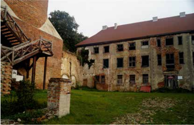
Fig. 3. Swobnica Castle. Reconstruction showing the position of the demolished west wall of the chapel and the line of its vaulting. The east wing on the right (remodelled) was added in the latter half of the 15th century (photo: K. Wroński)
