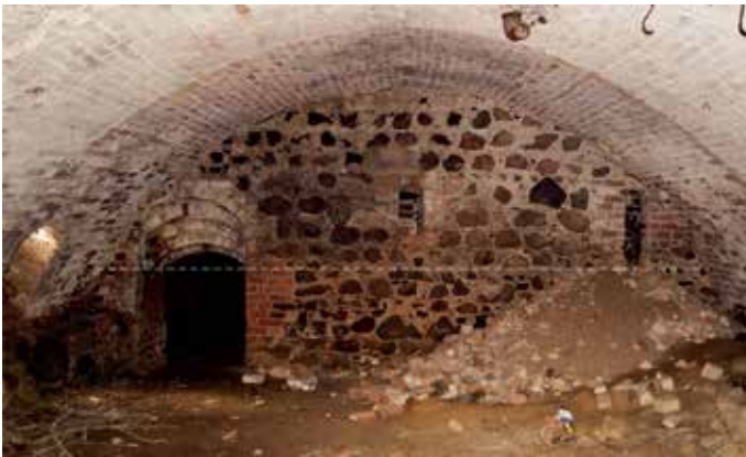
Fig. 4. South elevation of the undercroft below the former chapel at Swobnica (the dashed line approximates the original occupation level) (photo: K. Wroński)
