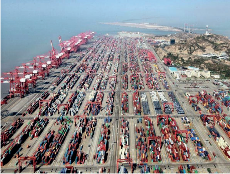
Figure 2. Yangshan Deep Water Port Source: (topchinatravel, 2018)
